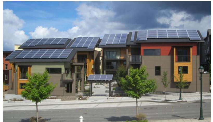
First community of all WaterSense labeled new homes in Issaquah, WA
