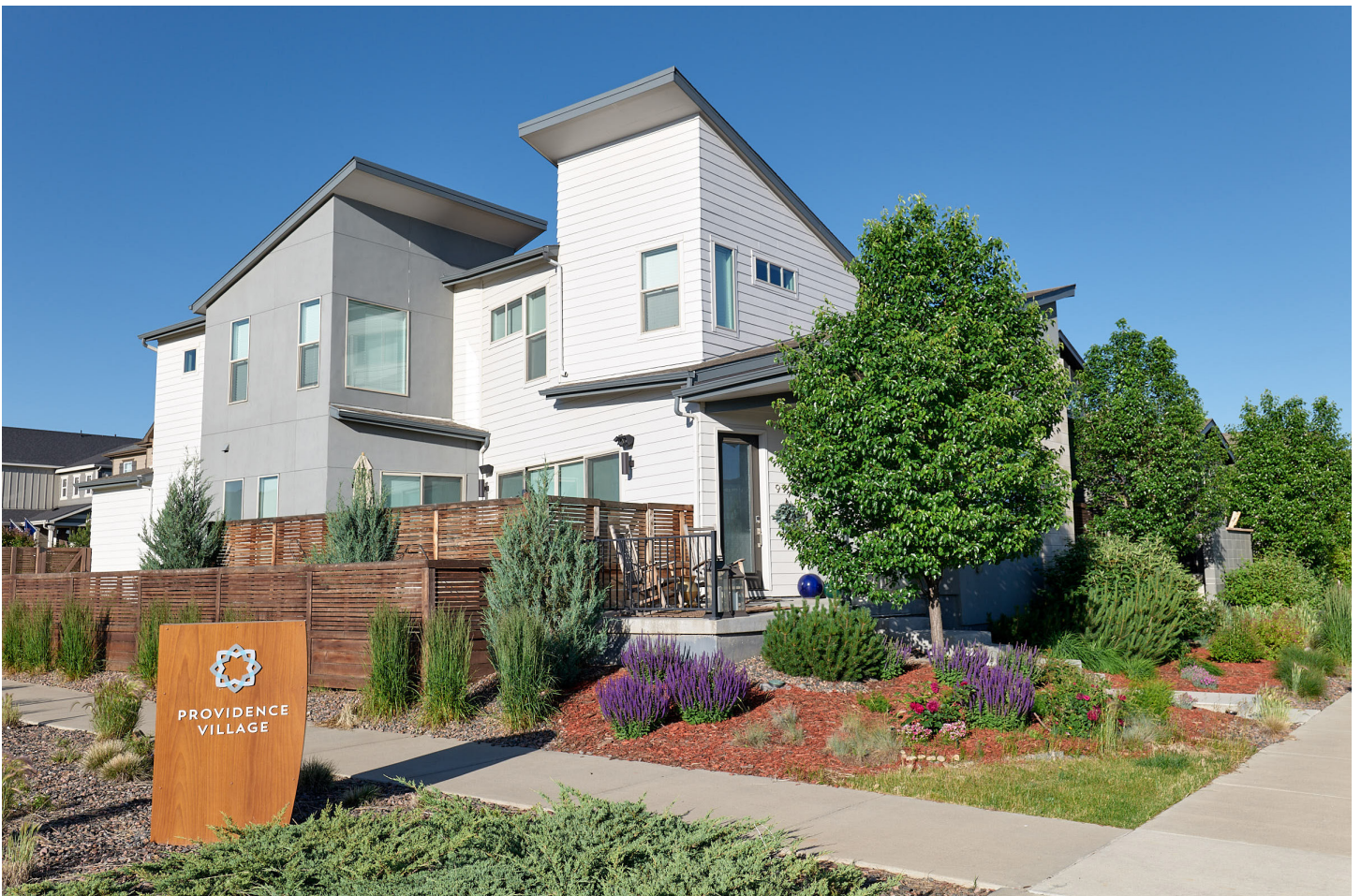
Homes in Sterling Ranch have dual water meters.
