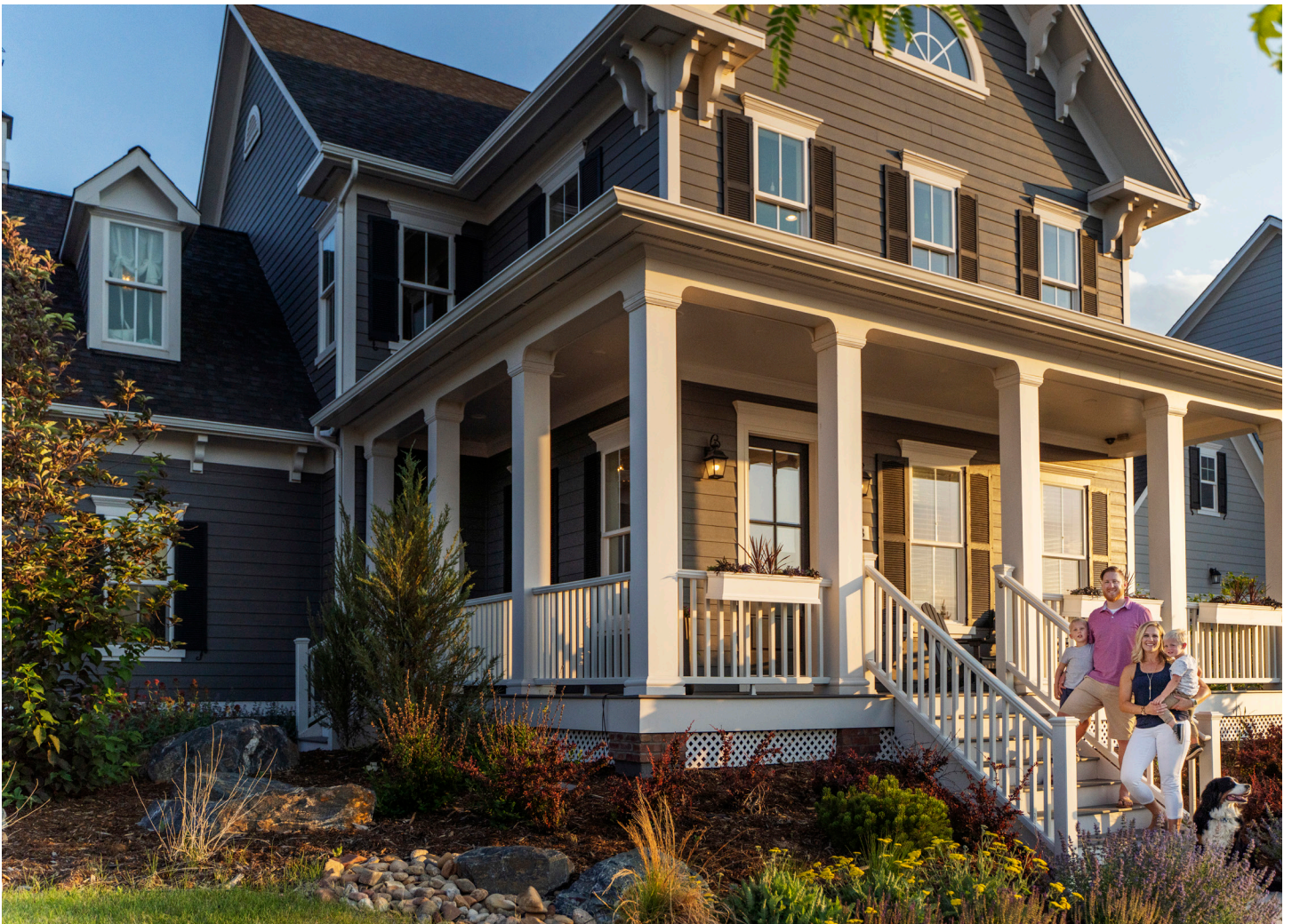
Homes in Sterling Ranch have dual water meters.
